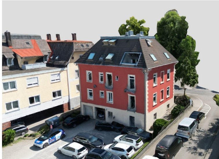
Figure 2.7: 3D textured model of a building created from a circular oblique flight via DJI Mavic Mini 3 Pro UAV.
