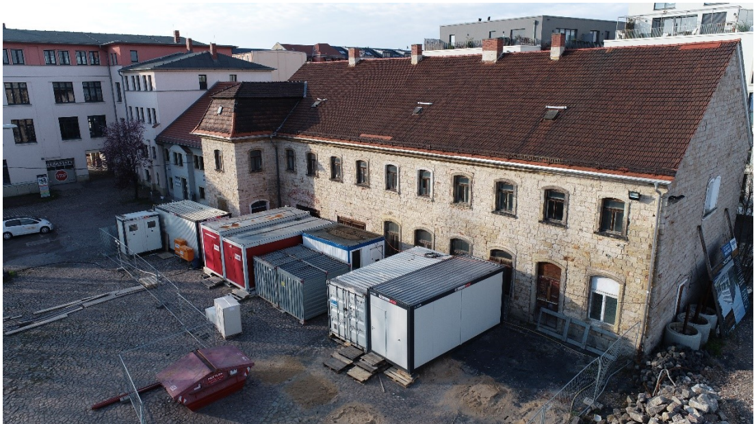
Figure B.8: Sample (2) of photograph captured by DJI Phantom 4 RTK on 09.04.2023.
