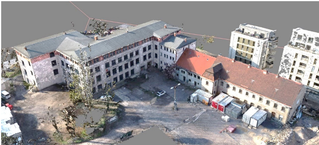
Figure 5.23: Dense point cloud created by using the data captured by the DJI Phantom 4 RTK.
