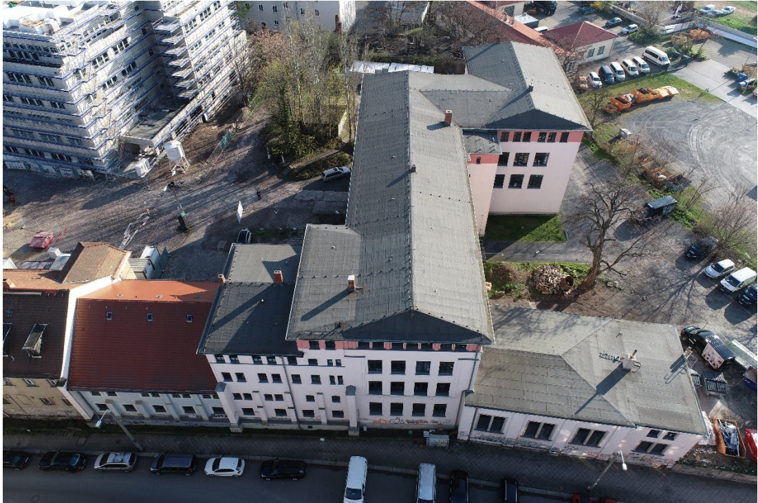
Figure B.7: Sample (1) of photograph captured by DJI Phantom 4 RTK on 09.04.2023.
