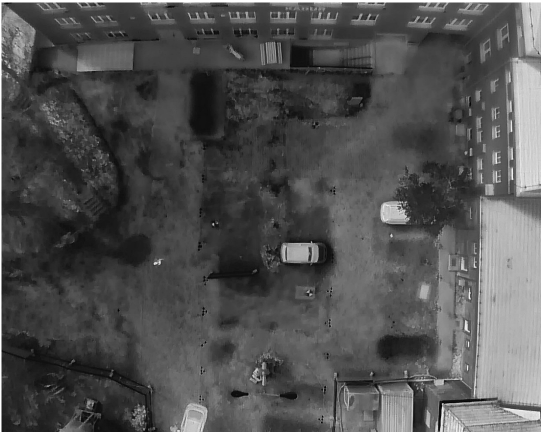
Figure B.10: Sample (2) of thermal photograph captured by DJI Matrice 30T on 13.04.2023.
